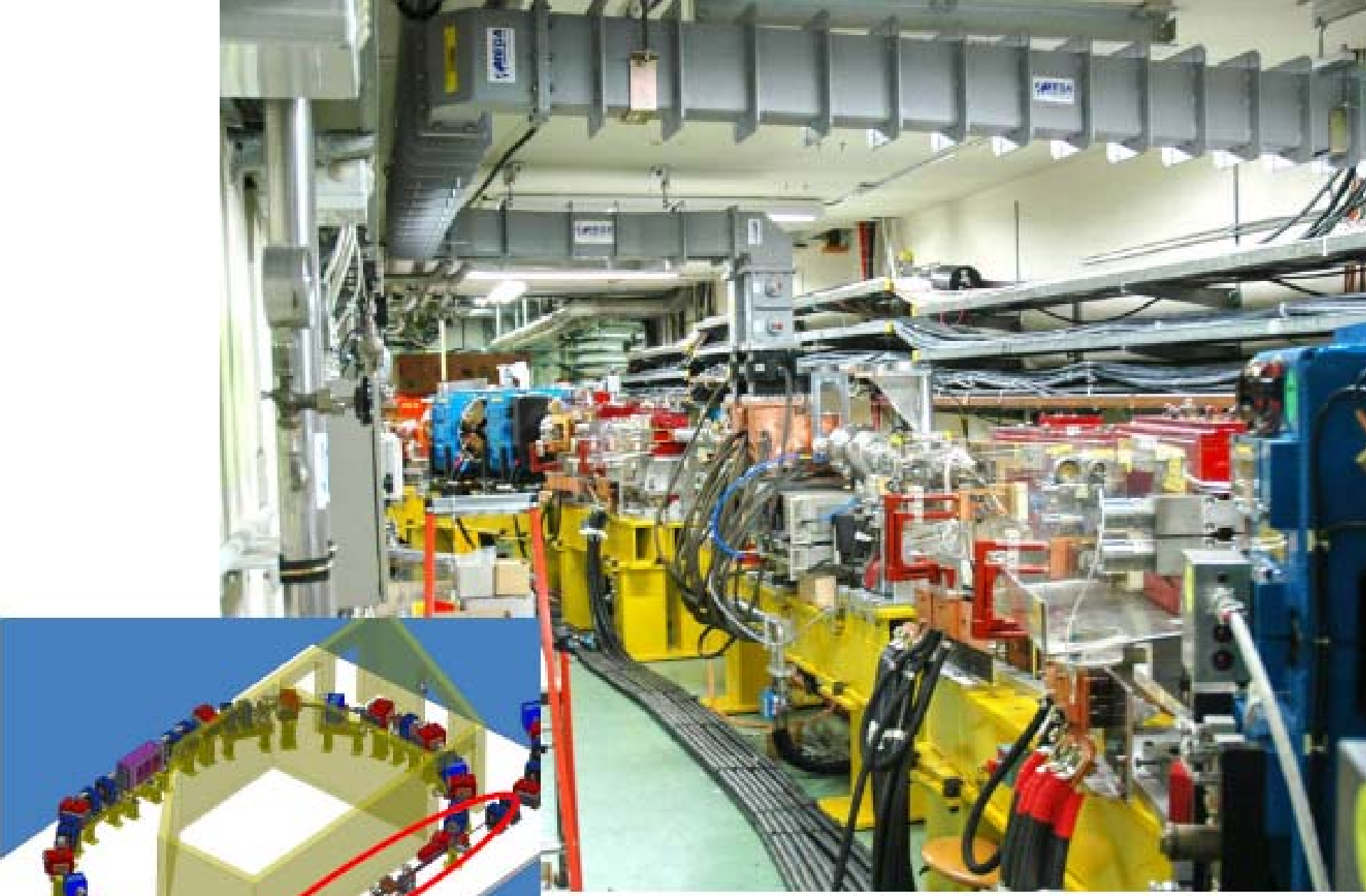
Delay Loop installation
